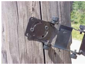
Mount sensor on backside of pole and allow room to pivot bracket in semi circle slot holes for final adjustment. (Model 1000V shown) Model 1000 no bracket with unit.
